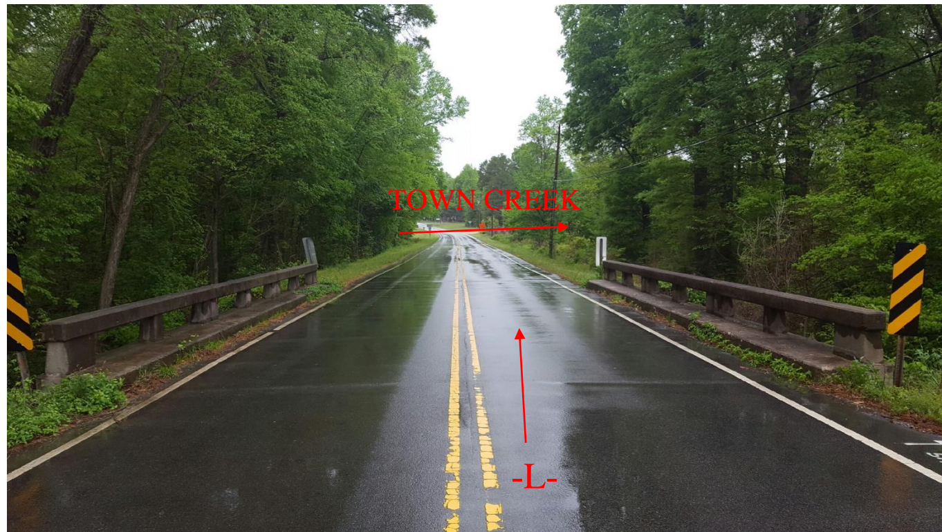
Photograph No. 1: At End Bent 2 looking towards End Bent 1
