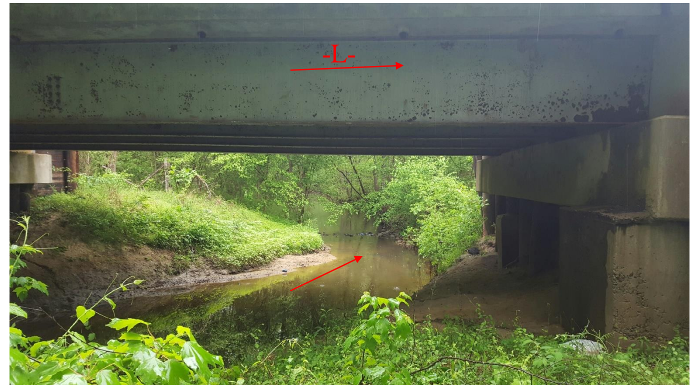
Photograph No. 2: Looking Downstream
